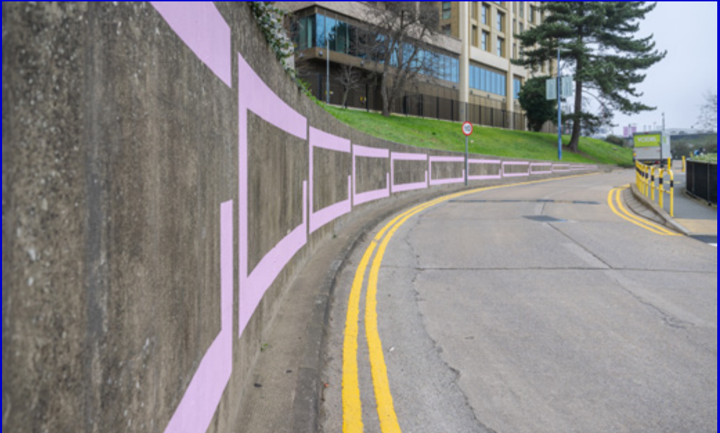
Above: Site entrance
