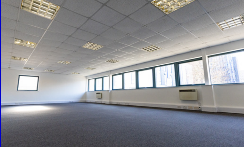
Above: Unit 1, office space
