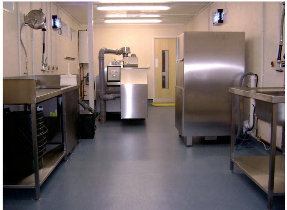
Food waste is first emptied from the waste collection bins on to the sorting table before being pushed into the hopper of the FWD. The captured dewatered waste is then loaded into the IVC. A utensil washer ensures the bins are kept clean.
