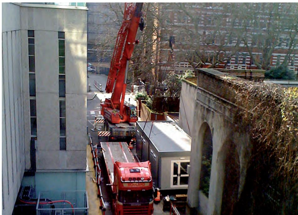
*The CompPod is delivered and craned into position requiring connection only to external mains services before being fully operational.*
