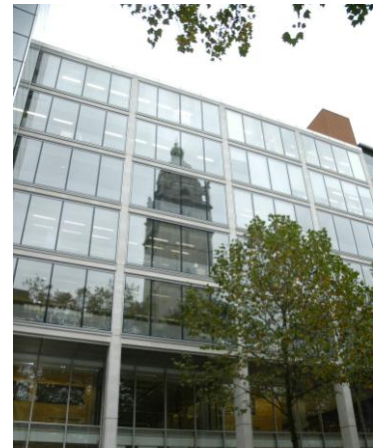
Sir Alexander Fleming Building
