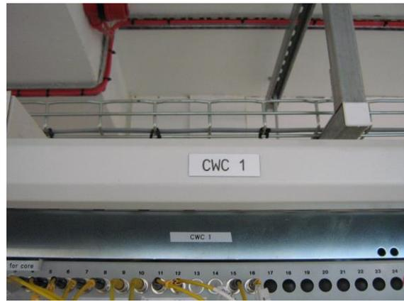
The picture on the left shows labelling done on the door with CWC ID and cabinet ID. The one on the right Shows CWC ID on the cabinet frame with 'traffolyte' type laser engraved label (only cabinet ID is missing).
