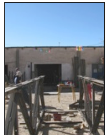
11th August The bridge takes shape!
