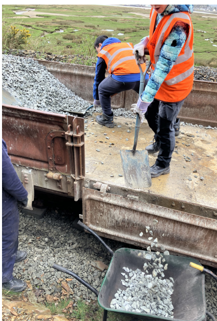
Ballasting the tracks
