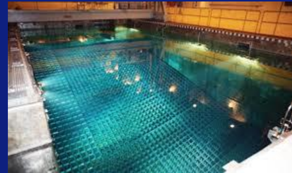
Spent Nuclear Fuel (SNF) storage pond.
