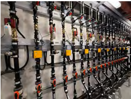
Manifold wall for optimized LC
