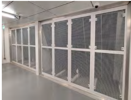
Fan coil wall coupled with different heat rejection options
